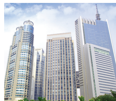
Building &amp; Rock Anchoring
