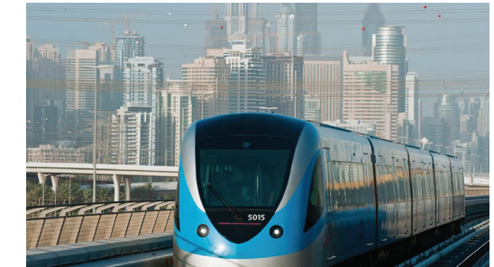
Dubai Metro Rail
